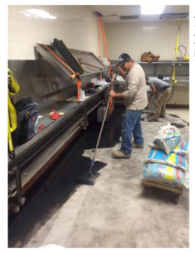
An Ardex Water Mitigation System was applied to completely eliminate any water issues and prevent leaks into the offices below.
