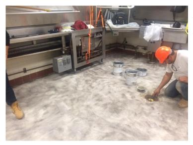
Ardex SDT product was then applied in order to level the floor flush to existing areas not receiving new floor and to ensure proper drainage to the existing drains.
